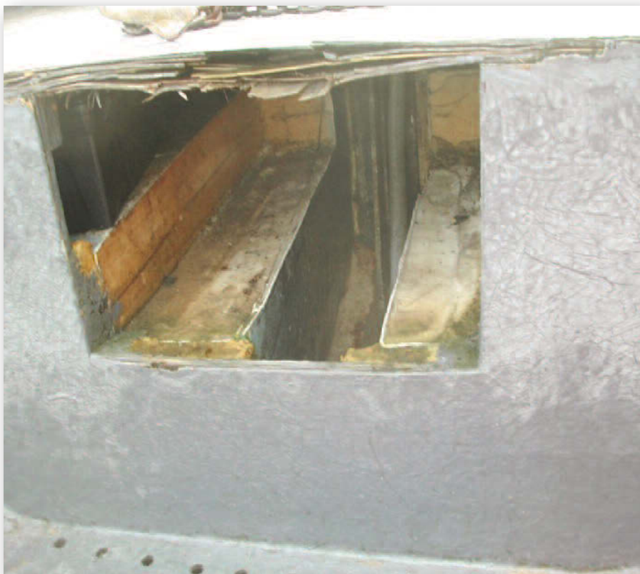
The cut away under the helmsman's seat showing delamination.
